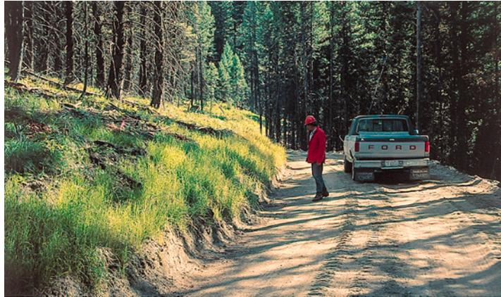
Grader damage to inside ditch toe slopes exposes an easily erodible surface and is a source of sediment.
