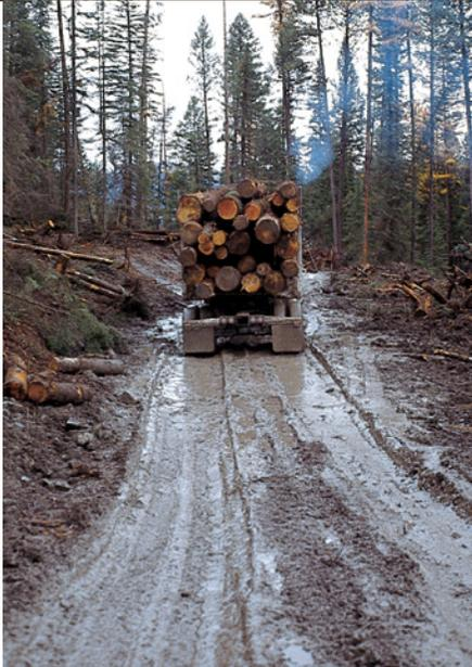
Roads receive heavy use during logging. Be aware of early signs of damage. Serious damage to road surfaces starts with excess water. Standing water is a sure sign of road-drainage problems. Ruts indicate that road strength is deteriorating.
