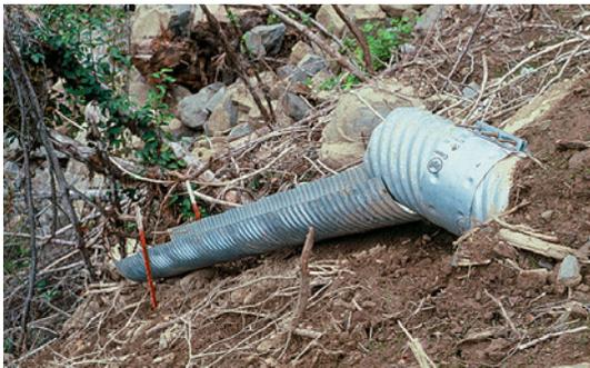
It may not always be possible to have the culvert extend beyond the fill. For steep fills, a half-round or flume should carry water beyond the fill.
