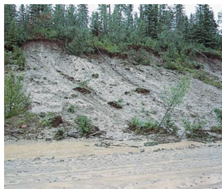
Poor road surface drainage caused this fill-slope erosion.
