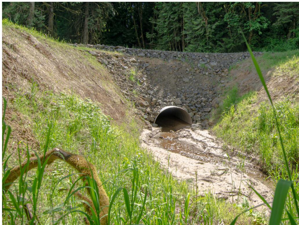
**Soil foundation.** Bedrock crossings may require bottomless arch culverts, bridges or fords.
