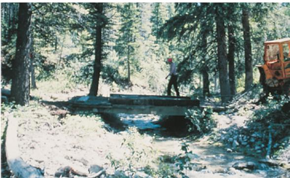
This 20-foot portable bridge was hauled on a flatbed truck and set into place in one day. The bridge cribbing that supports it is made from 10-foot-long timbers laid on the ground 4 feet from the stream bank.
