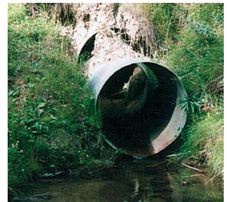
Watch for damaged culverts that need replacement. Repair work should be completed during dry weather.
