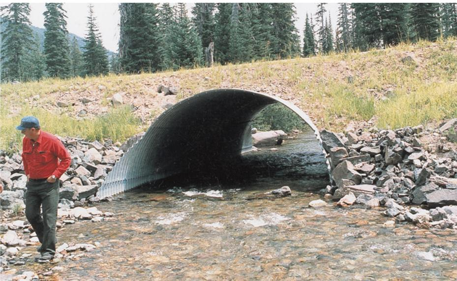
Bottomless arches leave the streambed intact, so fish can pass through easily. Natural streambed roughness creates pockets of low water velocity where fish can move more freely. Arch footings should be secured to bedrock to prevent the structure from failing.
