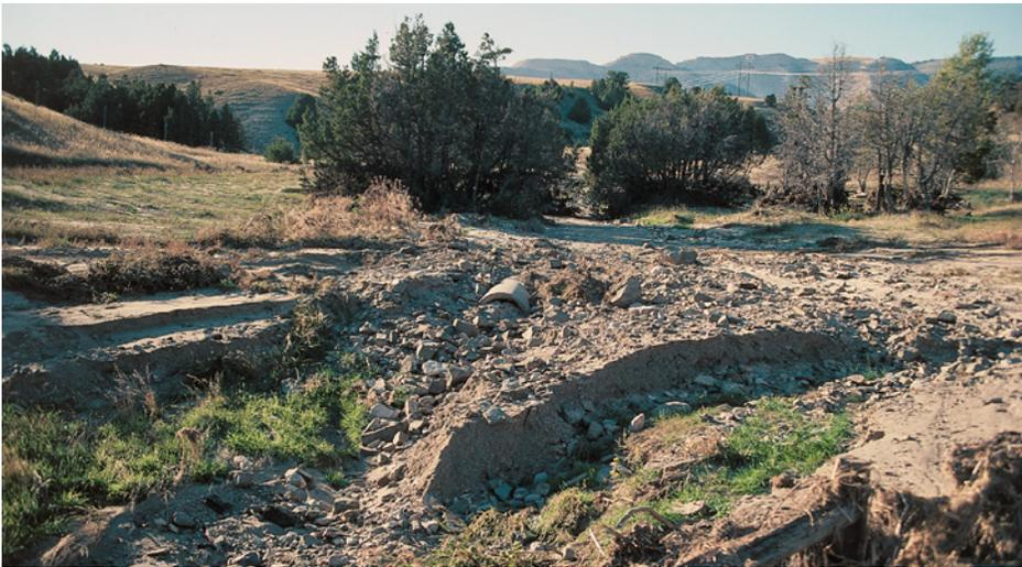
**Planning for a stream crossing must include considerations for potential flooding. When overlooked, the potential for water-quality damage is enormous. The costs of this plugged culvert road washout repair will far exceed the costs of a properly planned installation.**
