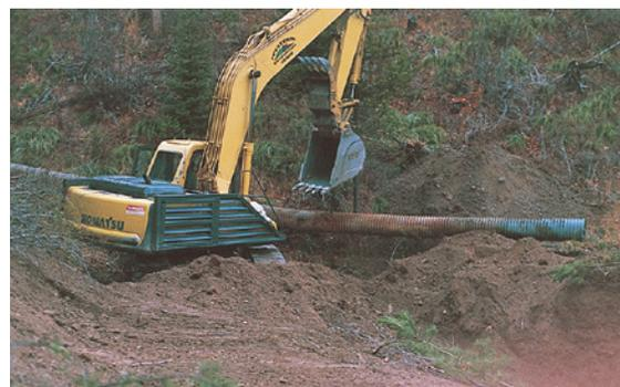
**When vacating a road, removal of all stream-crossing culverts and associated fill material is required. Non-drivable water bars (cross-ditches) should be installed to drain the road surface. Space water bars more closely, because with time they may fill with sediment.**
