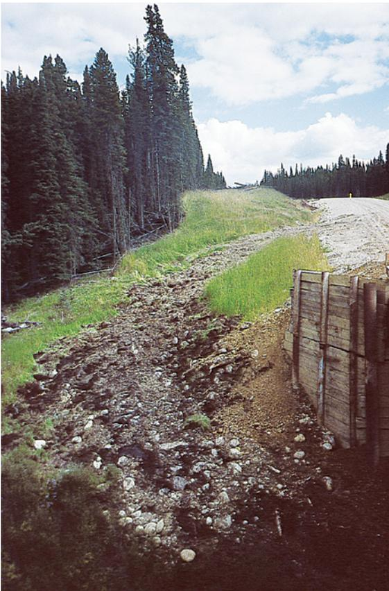
**Keep road drainage under control. Even with grass cover, runoff and sediment have flowed around this abutment and drained directly into the stream.**
