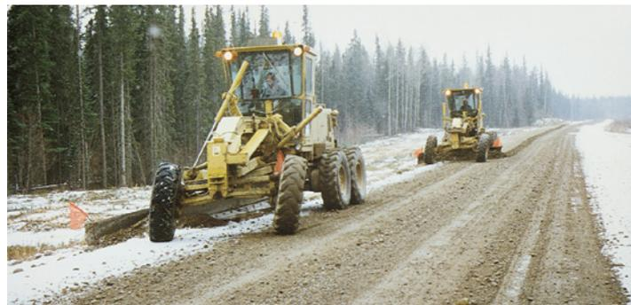
Slow, controlled grader operation is key to reducing culvert inlet and outlet damage. Reduce damage by keeping graders on the road running surface. Never side-cast gravel toward culvert inlets or outlets.
