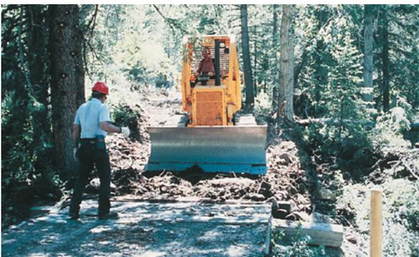
A small tractor built the road approaches to this temporary bridge. Over a three-week period, the bridge carried approximately 25 truckloads of logs.
