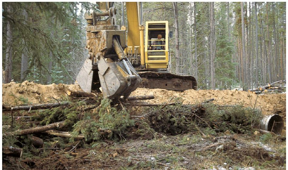
**Slash-filter windrows are made of compacted logging slash installed along the base of fill slopes during road construction. Built by excavators, these 3-by-3-foot barriers are very effective at slowing surface runoff and keeping sediment from entering streams.**
